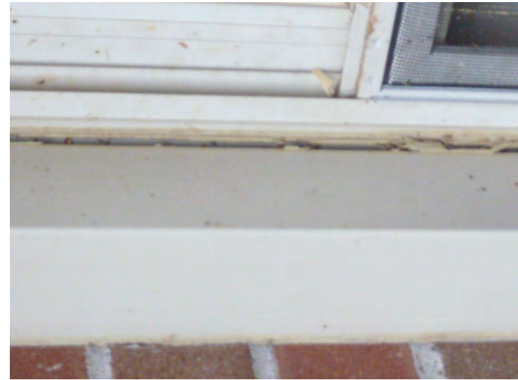
6. Caulking at windows and doors is failing in adhesion and is shown for replacement.
