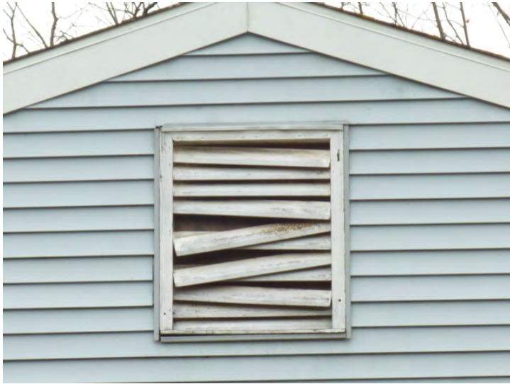
5. Fixed wood attic ventilation louvers are failing site-wide and are shown for replacement.
