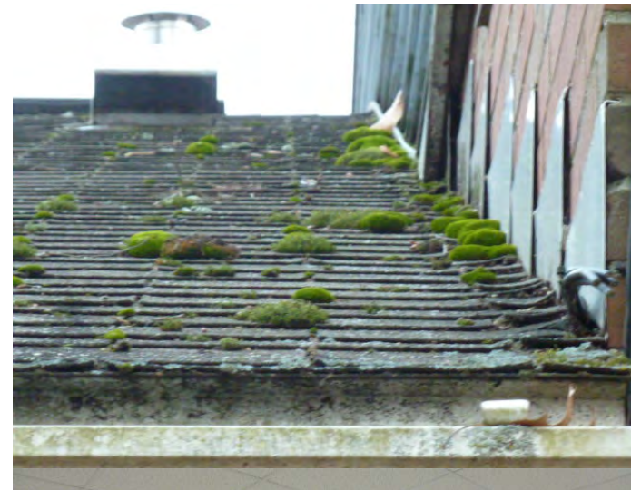
8. Extensive organic growth is present on north facing roofs and the granular surface of the shingles is decaying.
