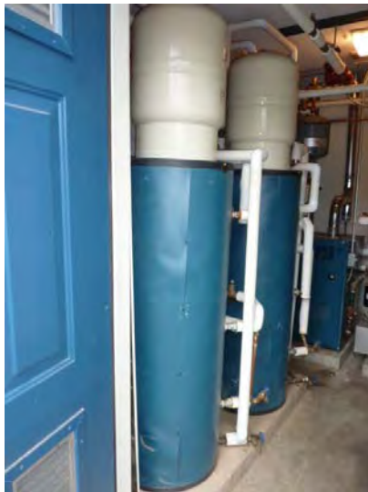
15. Typical unit level gas-fired Burnham boilers and hot water heaters are scheduled for replacement on normal cycles.
