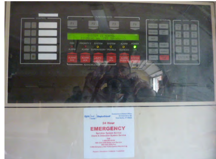
16. Fully addressable Simplex fire alarm panel monitors 4 slave panels around the site.
