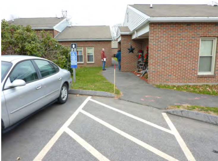
3. Asphalt paving at parking lots and walks is in good condition and shown for crack fill, sealcoat and replacement later in the term.
